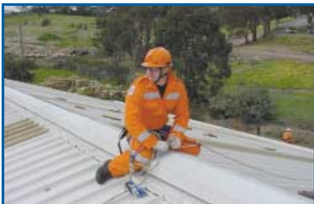
Roof-top safety system training, Mornington, March 2002.
